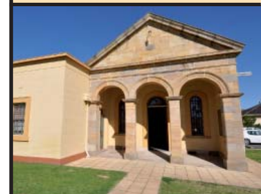
Court House - Wollongong
